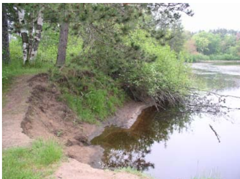
Streambank on the Dead River to be stabilized and restored using live fascine bundles and native plant seeds and plugs.
