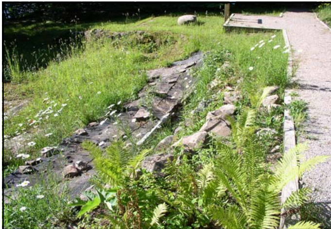
Stone Quarry restoration site covered in tar paper in order to eradicate weeds prior to planting
