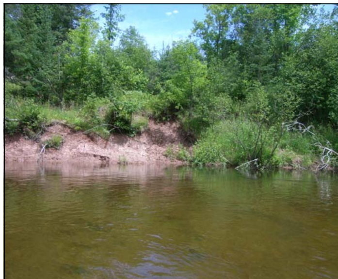
Eroded streambank on the Otter River.
