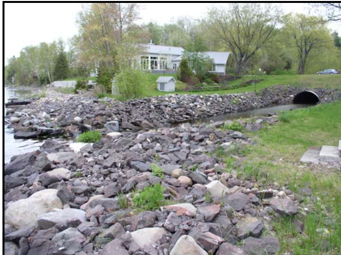
The stream crossing at Zeba Creek was remediated with a new arched culvert with a natural bottom designed for fish passage and rock armoring of the creek's outlet below the culvert which dramatically curtailed erosion.
